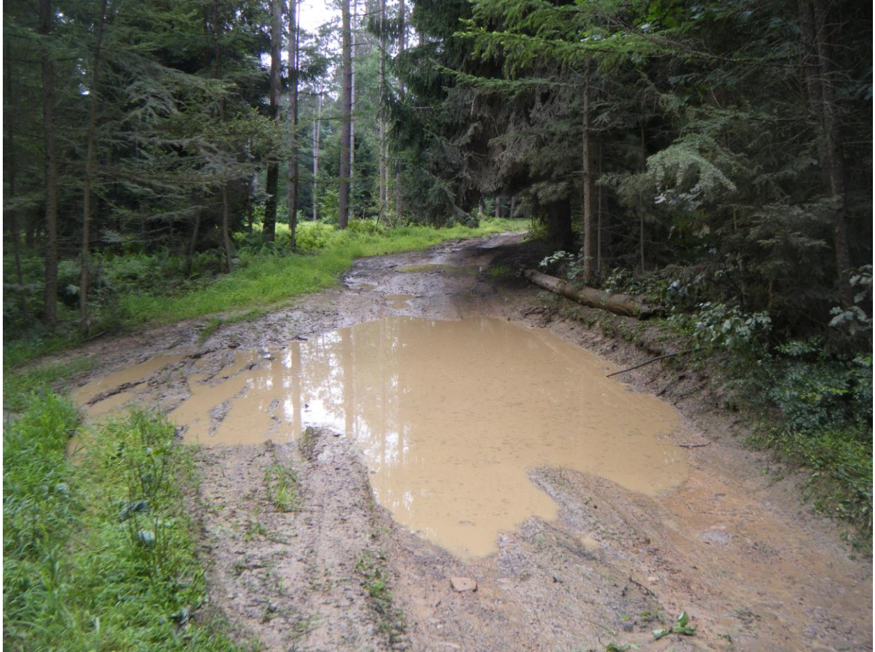
Fig.4 Two foot deep mud holes
